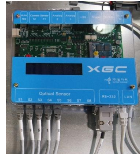
Labeling for Cables
